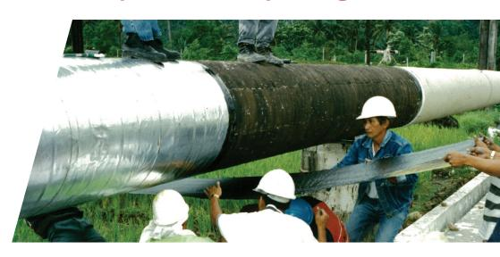
An All Purpose, Weatherproofing and UV Resistant Membrane for Exposed and Buried Pipes **PROTECTO SEAL 50 BUTYL** is a cold applied, self-adhering membrane composed of a 50 mil, self-adhered, butyl based, waterproofing membrane with a tough cross laminated polyethylene film laminated to an aluminum foil for UV resistance as well as weatherability.
