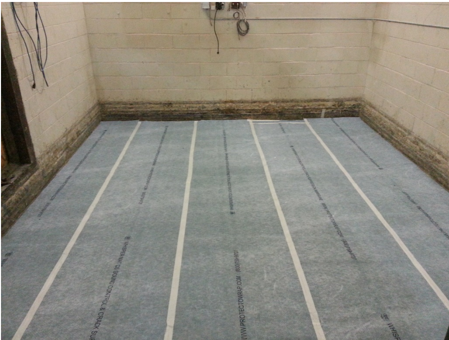
Figure 2 – Underlayment installed on the concrete slab.
