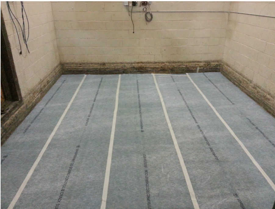
Figure 2 – Underlayment installed on the concrete slab.
