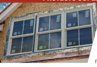
A high performance window and door flashing tape designed to be applied down to -20°F (-28.88°C) without the use of primer or mechanical fasteners on most substrates. Provides a full 12 month UV exposure and contains no rubberized asphalt.
