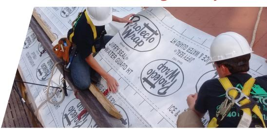
A premium high temperature, 25 mil self adhered roof underlayment Jiffy Seal Ice & Water Guard HT 25 is a cold applied, self-adhering membrane composed of a proprietary slip resistant, tri-layer, woven polypropylene fabric coated on one side with a layer of rubberized asphalt adhesive.
