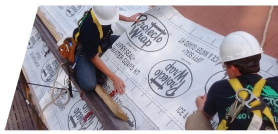
A premium high temperature, 25 mil self adhered roof underlayment Jiffy Seal Ice & Water Guard HT 25 is a cold applied, self-adhering membrane composed of a proprietary slip resistant, tri-layer, woven polypropylene fabric coated on one side with a layer of rubberized asphalt adhesive.
