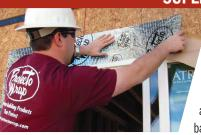
A high tack, tenacious, durable, self-adhered air/vapor barrier tape system used for sealing PVC and aluminum fin windows and doors; window and door openings; and as a full coverage air vapor barrier membrane.
