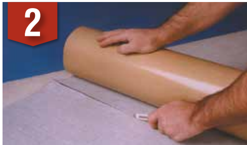
CUT MEMBRANE TO LENGTH
