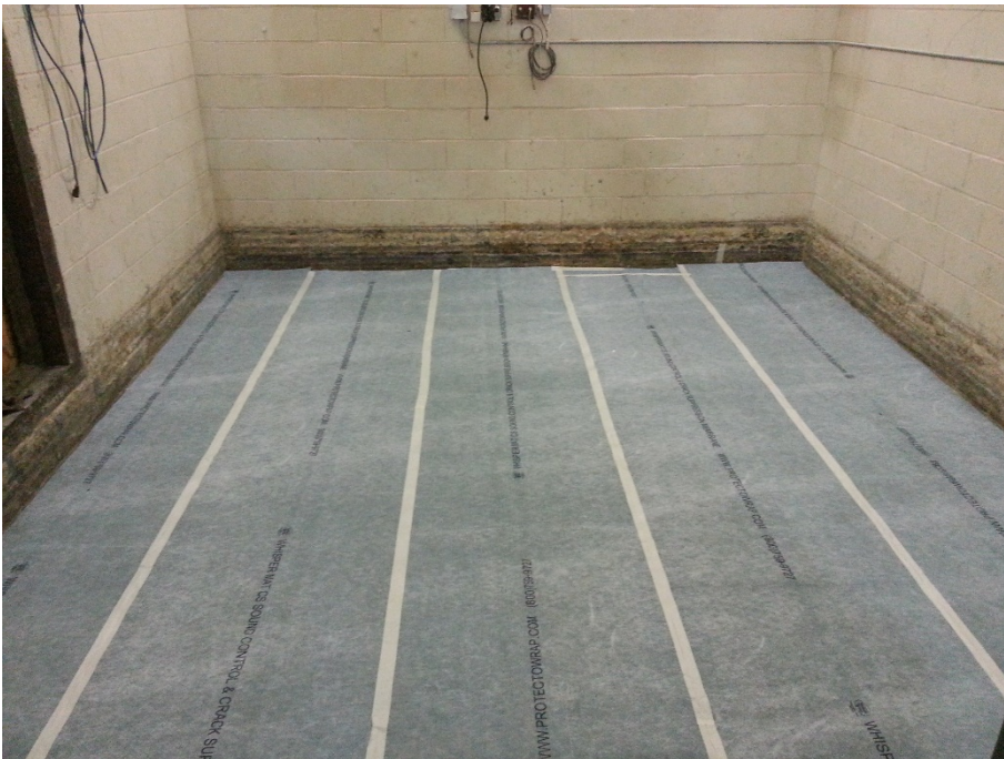
Figure 2 – Underlayment installed on the concrete slab.
