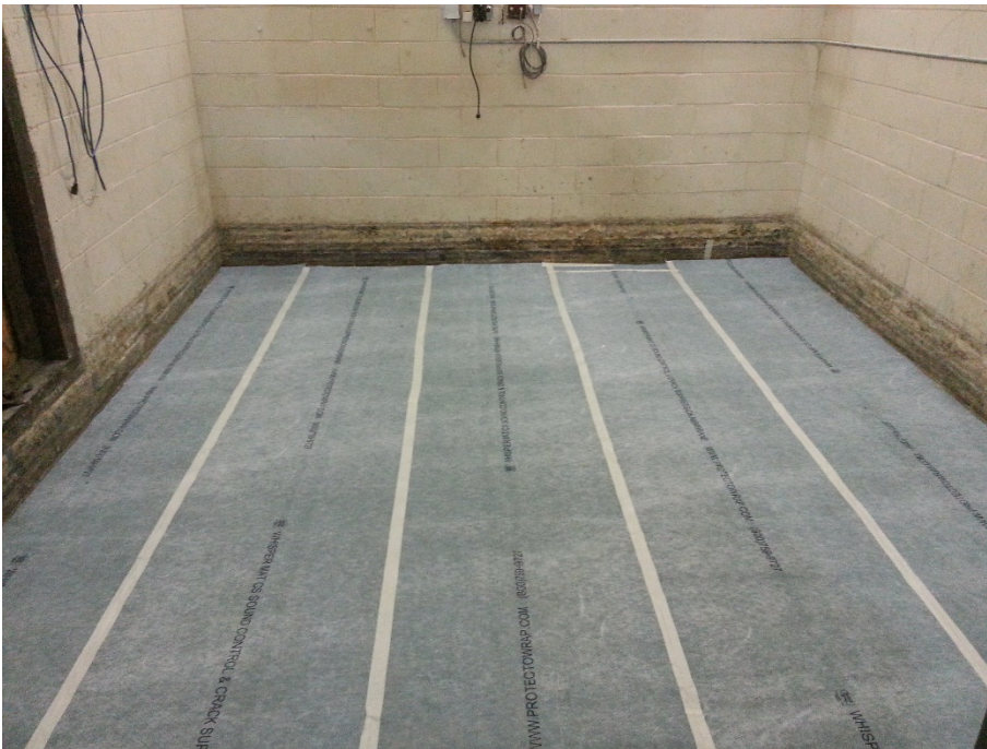
Figure 2 – Underlayment installed on the concrete slab.
