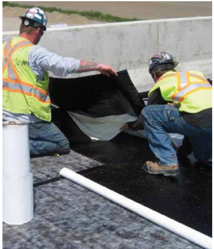
Silicone coated release film on the bottom allows the membrane to be easily positioned on the deck.
