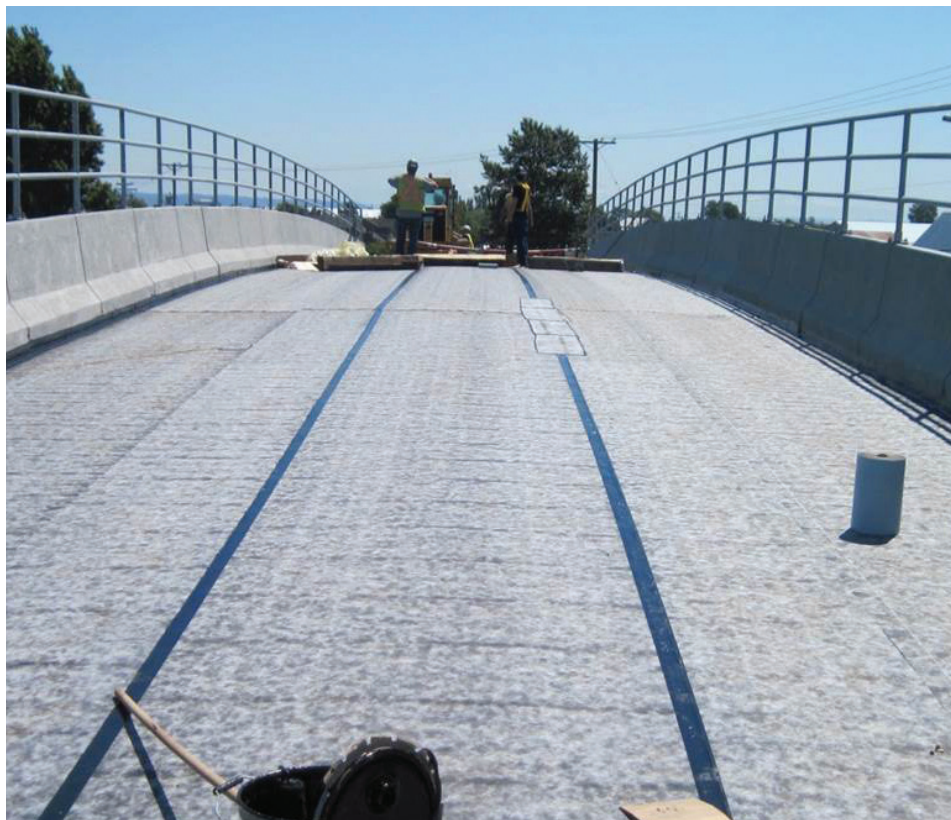
M-400A(R) rolls provide unique salvage edge (black SBS adhesive top) ensuring all roll laps are mastic to mastic cohesive bond for fully monolithic deck result.
