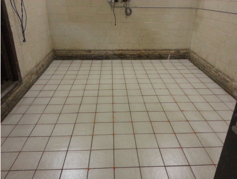
Figure 1 – Specimen mounted on the concrete slab. (Note: spacers were still present at the time the photo was taken, but were removed before installation of grout)
