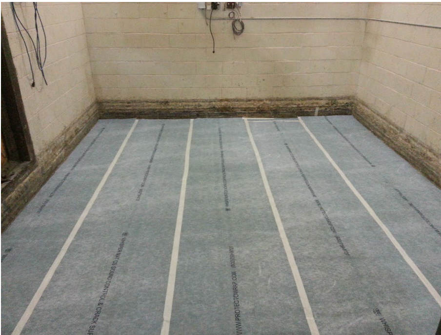
Figure 2 – Underlayment installed on the concrete slab.
