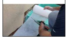
Apply liberal coat of Protecto LM Liquid Membrane to all overlap seams and ensure any exposed Protecto LM Reinforcing Fabric is coated
