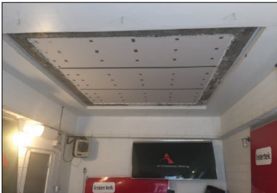
Receive Room View of Test Specimen Installation
