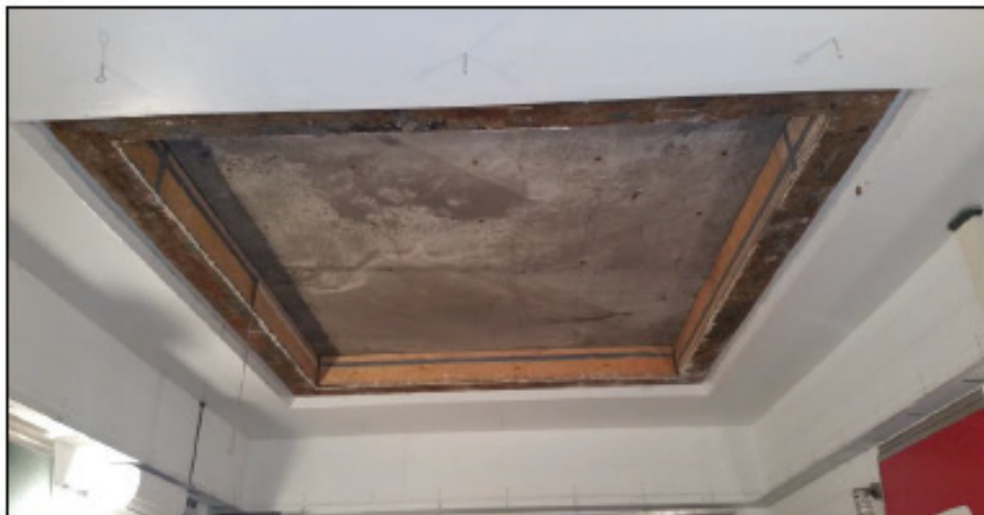
Receive Room View of Test Specimen Installation
