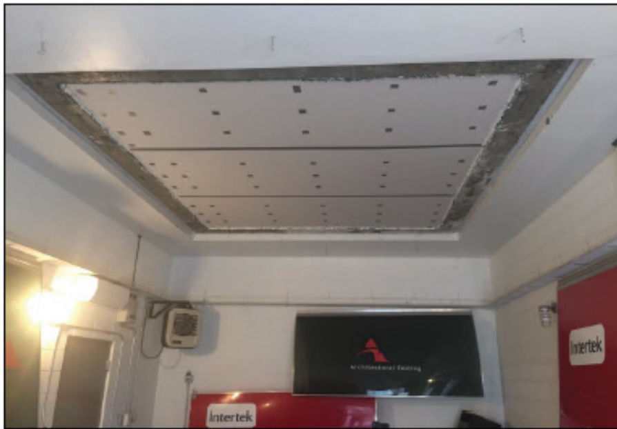
Receive Room View of Test Specimen Installation
