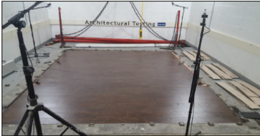
Source Room View of Test Specimen Installation
