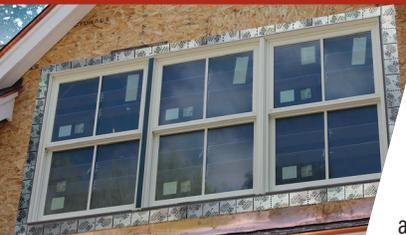
A high performance window and door flashing tape designed to be applied down to -20°F (-28.88°C) without the use of primer or mechanical fasteners on most substrates. Provides a full 12 month UV exposure and contains no rubberized asphalt.
