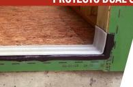
Its unique flange acts like a gasket, sealing off the sub-floor and preventing air and moisture infiltration under the threshold. Helps keep the door frame from racking and the sub-floor from swelling and warping.
