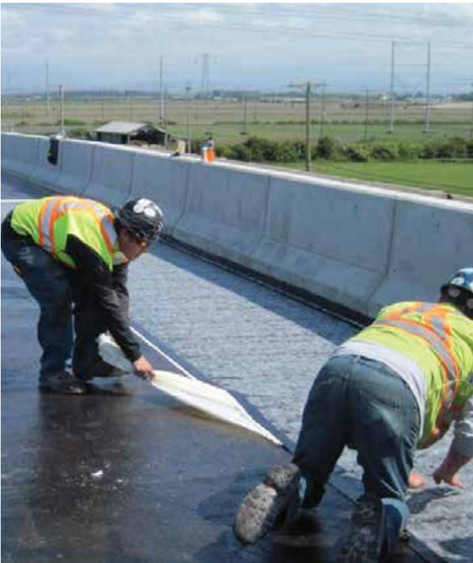
Release film removes easily after positioning membrane on overlap.
