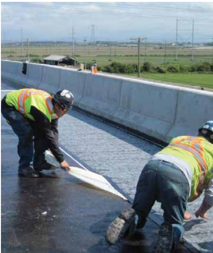
Release film removes easily after positioning membrane on overlap.
