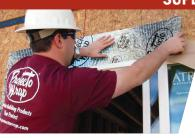
A high tack, tenacious, durable, self-adhered air/vapor barrier tape system used for sealing PVC and aluminum fin windows and doors; window and door openings; and as a full coverage air vapor barrier membrane.
